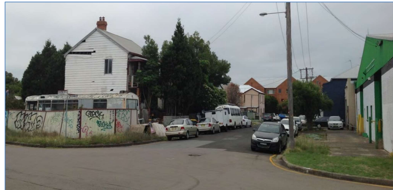
Figure 10 Buildings at the end of their lifecycle identified as likely for future redevelopment.
