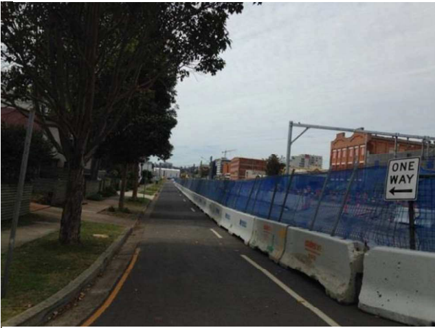
Photo 1: Station St looking east from Railway St
