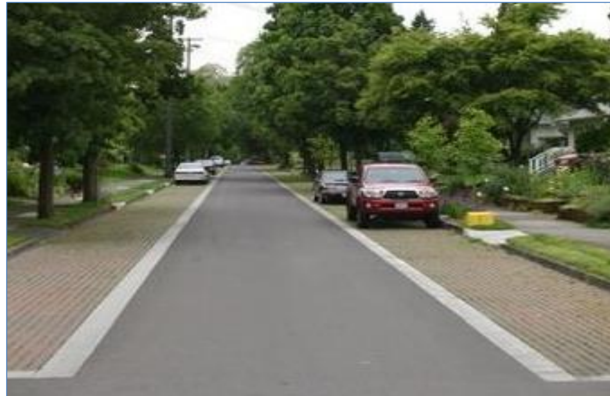
Figure 35 -An example of pervious paving applied to define on-street car-parking areas and facilitate stormwater management.
