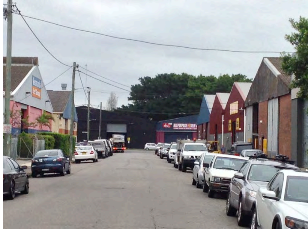
Photo 1: Part of Throsby Street characterised by gabled industrial buildings
