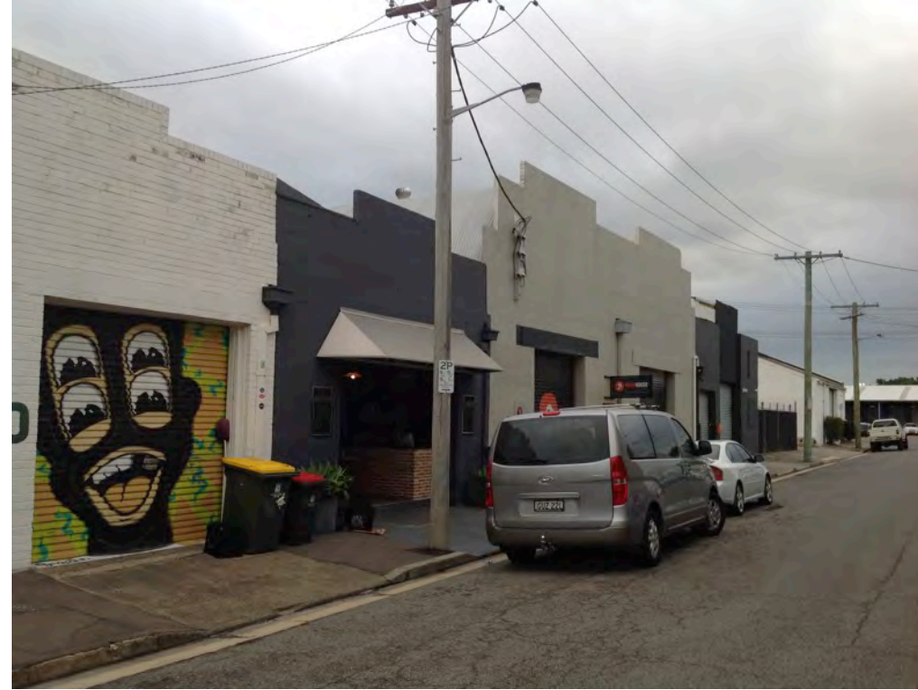
Photo 2 - Emerging industries quarter could evolve from existing industrial character
